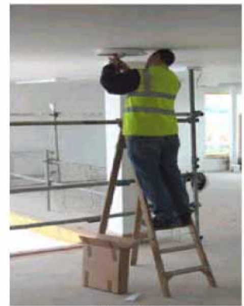
Correct use: Ladder right length, facing work
